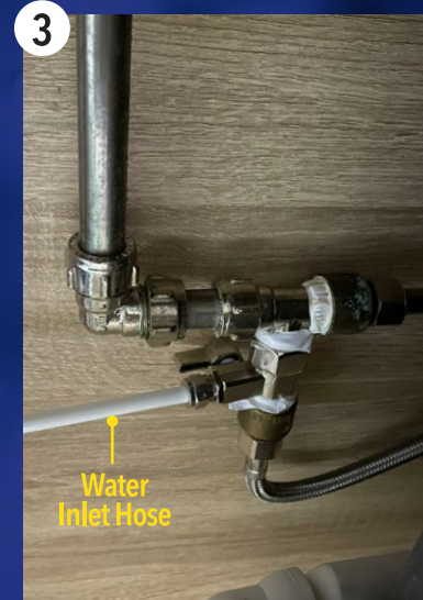
Set Up Water Inlet Hose Via Direct Pipe-in
