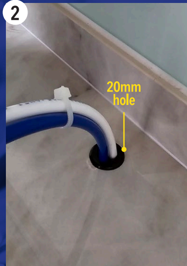
Drill A 20 mm Hole On The Counter Top For Water Inlet And Outlet Hoses
