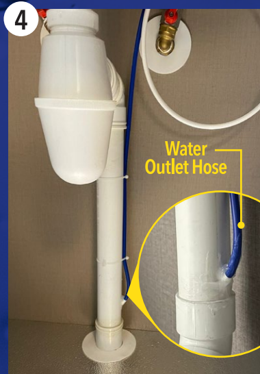
Water Outlet Hose Connect To Drainage Pipe
