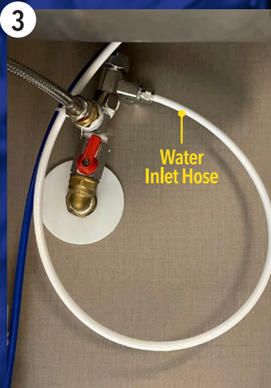
Set Up Water Inlet Hose Via Direct Pipe-in
